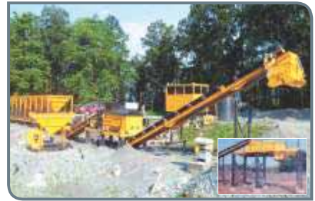
SOIL STABILISATION (WET MIX) PLANT
